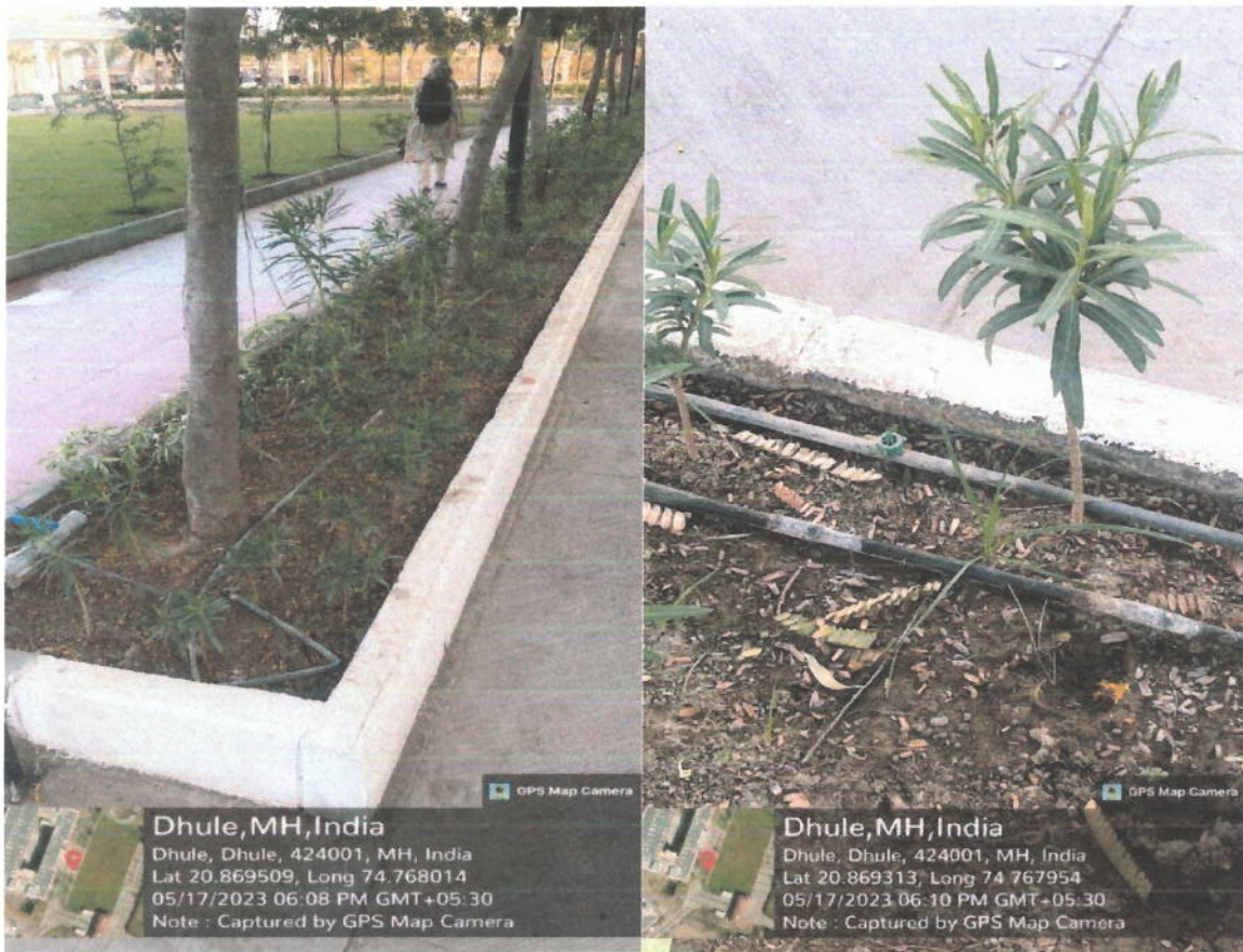
Photo of to decrease water consumption, drip irrigation system are used.
